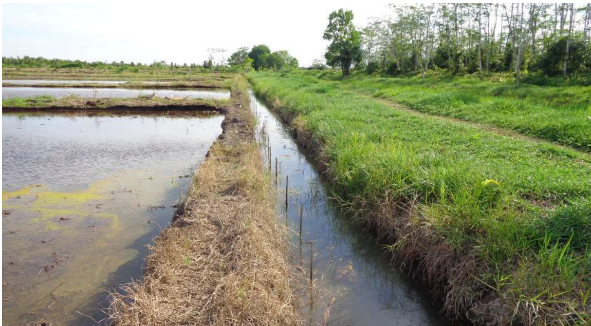
Gambar : Kondisi Saluran Pengairan lahan pertanian Desa Talio Hulu. / Condition of farmland irrigation channel in Talio Hulu Village.
