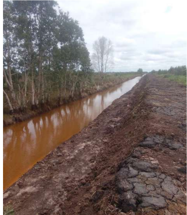
Gambar : Kondisi kanal yang telah direhabilitasi. Air tampak berwarna coklat kekuningan akibat kondisi pirit yang terekspos. / Condition of the rehabilitated canal. The water color is yellowish brown due to the exposed pyrite.
