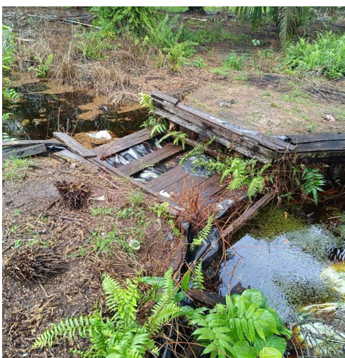
BRGM canal blocks in damaged condition found in (left) PHU Pulau Rupal and (right) Sungai Rokan–Sungai Siak Kecil PHU, Riau Province.
