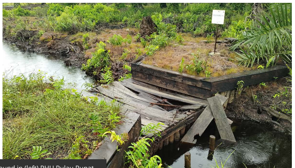
BRGM canal blocks in damaged condition found in (left) PHU Pulau Rupal and (right) Sungai Rokan–Sungai Siak Kecil PHU, Riau Province.
