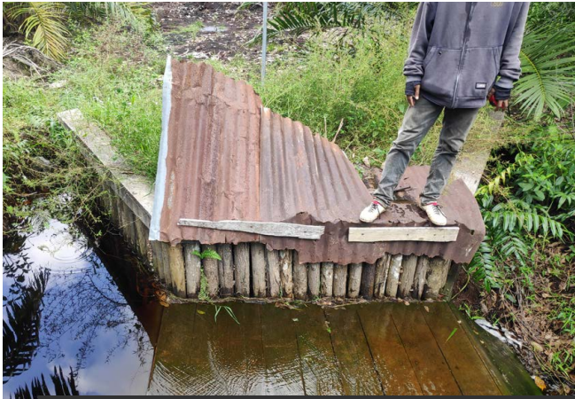
Canal blocks in Krueng Bubon–Krueng Meureubo PHU, Aceh Province: (left) in good condition and (right) overgrown with shrubs.
